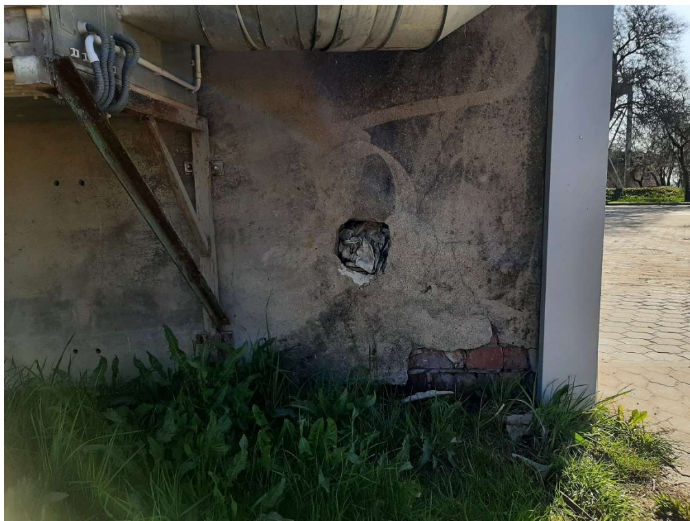
Att.5 - Fasādes remonts
